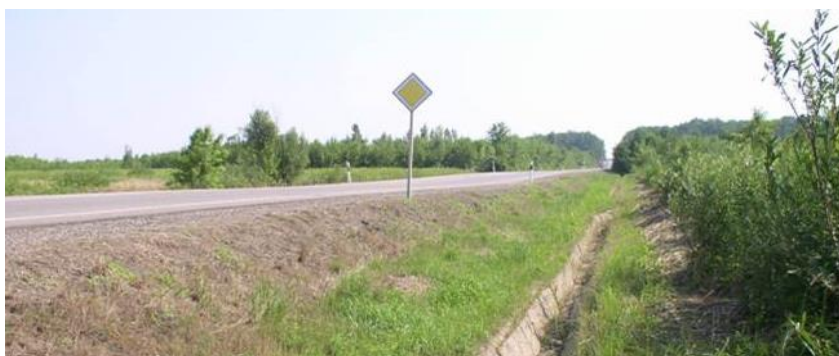
Figure 2 — Completed fly ash embankment in a Hungarian motorway M35
