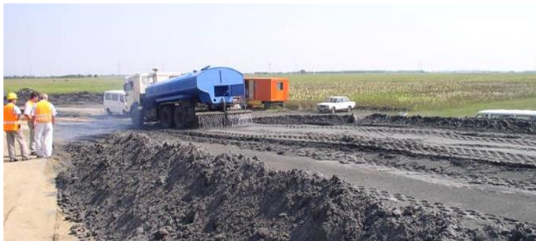
Figure 1 — Construction of fly ash embankment in a Hungarian motorway M35
